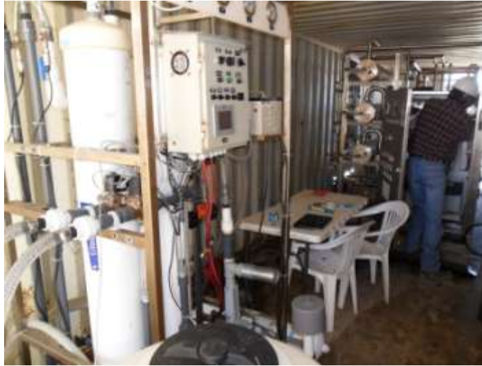
Figure 5: Picture of the hollow fiber, spiral wound and RO filtration systems
