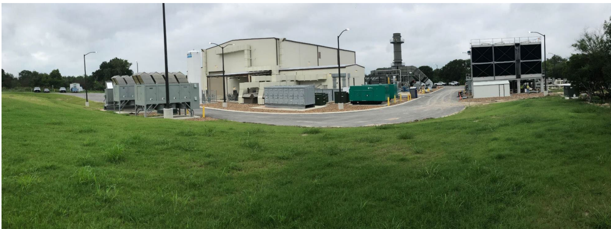
Figure 2a: STEP facility building (middle), cooling towers (right), heater and stack (middle), load banks (left)
