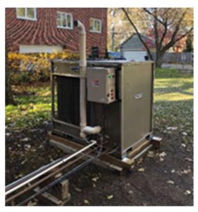
Figure 21: Example Natural Gas Heat Pump
