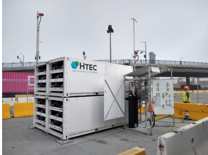
Figure 18 - Fueler installed at TraPac Facility
