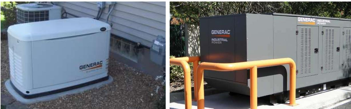
Figure 55: Example Residential and Commercial/Industrial Natural Gas Generator Sets
