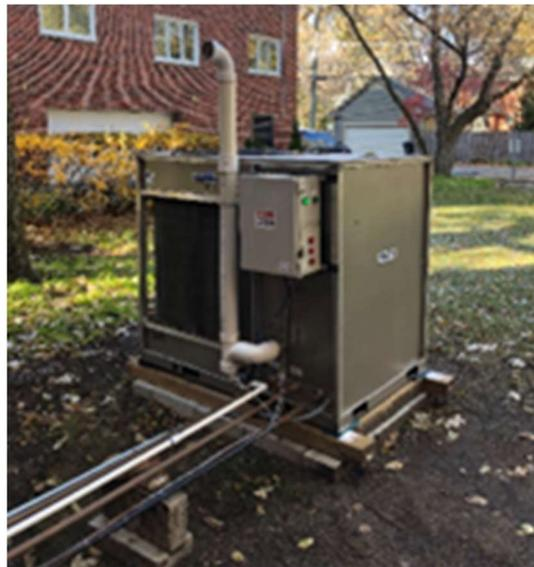
Figure 21: Example Natural Gas Heat Pump
