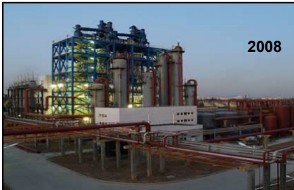
2 x 400 ton per day U-GAS® in Zao Zhuang City, China using coal
