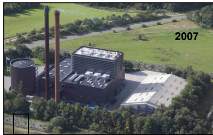
150 ton per day CHP Plant in Skive, Denmark using wood
