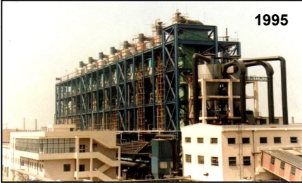
800 ton per day U-GAS® coal gasification plant in Shanghai, China
