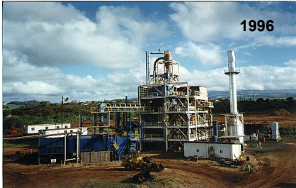
100 ton per day RENUGAS® demo plant in Maui using bagasse
