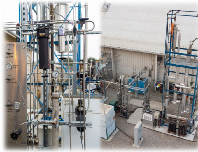
Upgraded 2-stage separator
