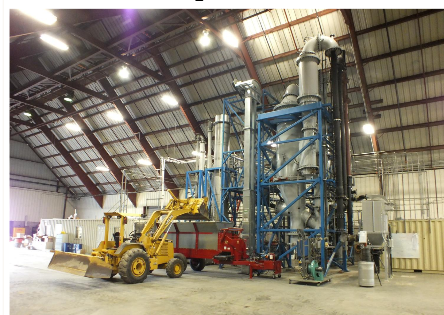
Fig. 1: Pilot-scale FICFB Gasifier at West Biofuels
