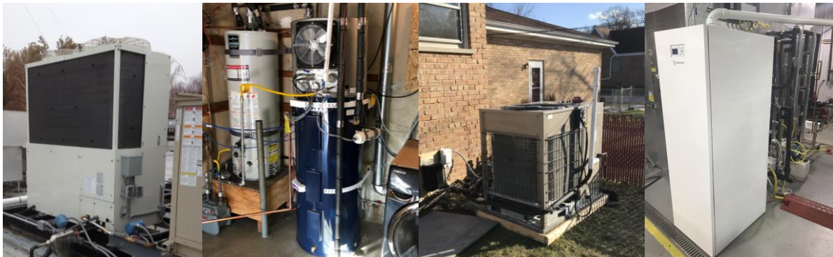
Figure 2: Commercial/Prototype THPs in GTI Demonstrations: Engine-driven VRF, Sorption-type Water Heater, Sorption-type Whole House Combi System, and Thermal Compression-type Heat Pump Boiler (Source: GTI)
