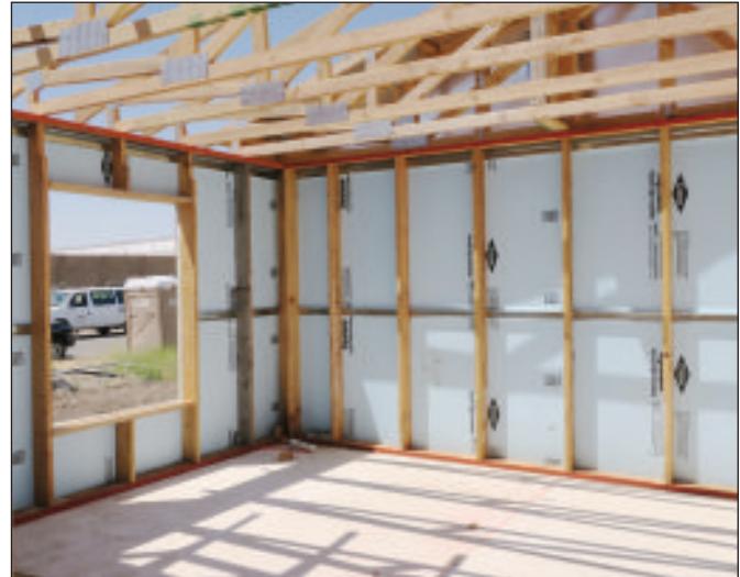
Fig. 6.8 Clear cavities for fast and uncompressed installation of low-cost, high-performance batt insulation
