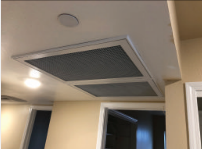
Fig. 7.8 Large air grill holds MERV 13 filters
