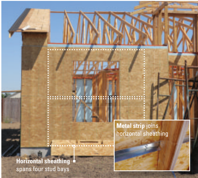
Fig. 5.10 Horizontal sheathing joined by metal strips The assembly was developed at Dream Creek by George Koertzen, the project designer and its construction manager.
