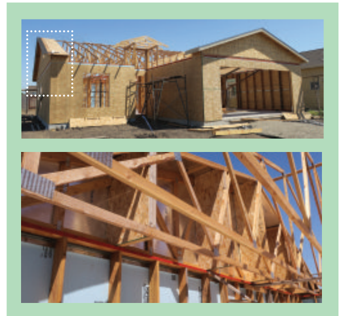
Fig. 5.11 Pre-assembled gable-end truss - lifted as a single piece
