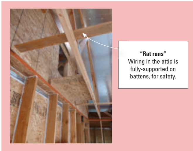
Fig. 9.5 Attic wiring is fully-supported, protected and easy to find Wire in the attic is fully-supported by what George calls “rat runs:” 1” x 4” or 1” x 6” lumber that crosses and connects the joists or trusses. With that support, there’s less risk that workers will accidentally snag and pull a wire during construction or later, after the wiring is buried under insulation.
