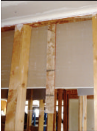
Fig 6.16 Wall board connected with OSB splice strips
