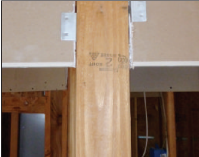
Fig. 6.7 Drywall clips in place of extra studs
