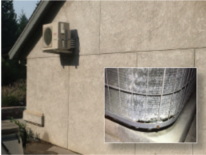
Fig. 7.6 Ducted mini-split outdoor unit mounted high on the wall Keeping the outdoor unit high on the wall helps limit the amount of dust, grass and leaves that might otherwise clog the coil and reduce AC and heating capacity. (It also avoids the problem of dog urine..!)
