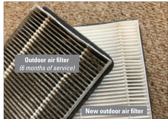
Fig. 10.3 Used v. new outdoor air filters from an ERV
