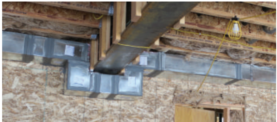
Fig. 3.9 Don't do this! Big energy waste. The architectural decision to use a deep beam forced the HVAC duct to make four right-angle turns. That decision multiplied the air flow resistance of these three feet of duct by a factor of 100.
