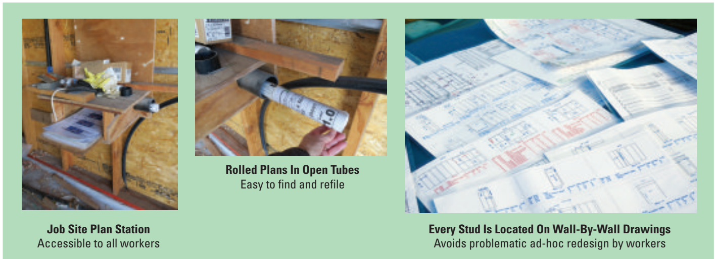
Fig. 4.2 Full set of plastic-laminated detailed drawings—on-site and accessible to all workers—reduces confusion and speeds completion
