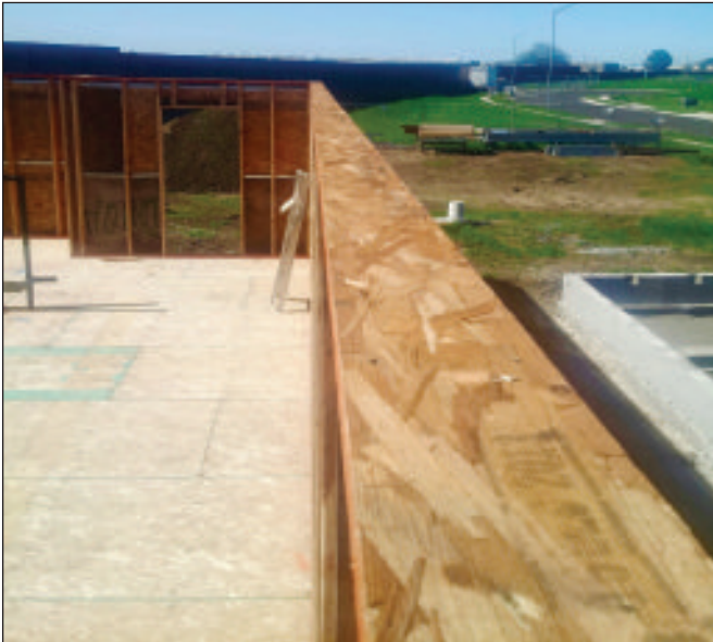
Fig. 6.3 Single top plate
