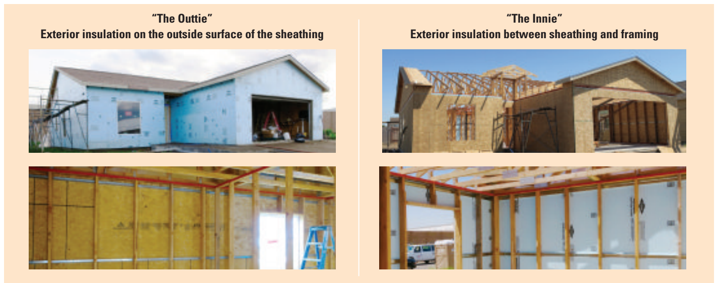
Fig. 5.16 Exterior insulation layer—two alternatives
