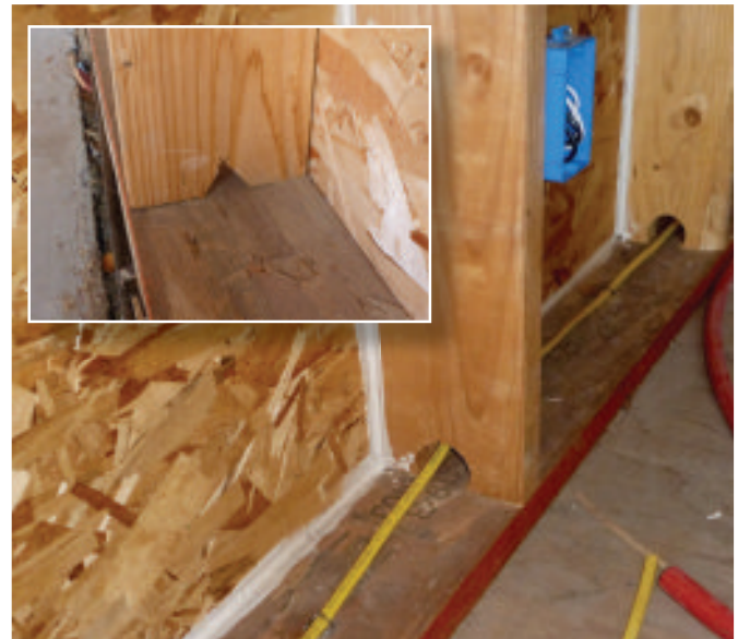
Fig. 5.9 Notches for wiring, cut into the base of exterior studs Avoids crushing or squeezing insulation with mid-cavity wiring.
