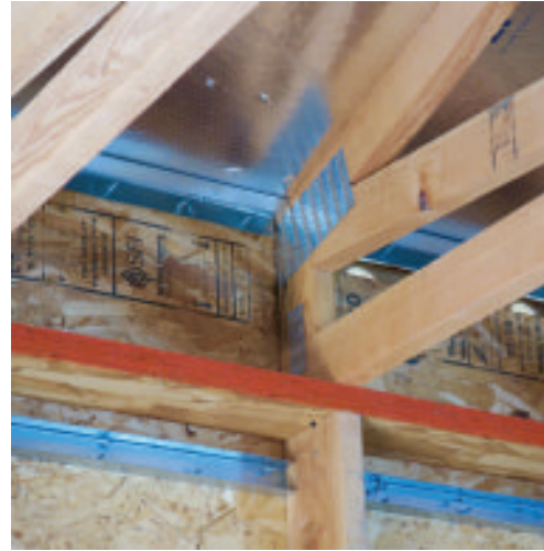
Fig 6.13 Raised heel truss
