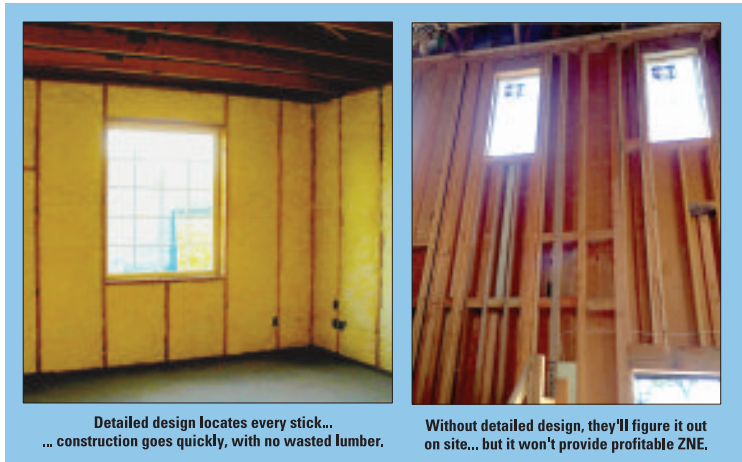
Fig. 5.3 Detailed design avoids waste
