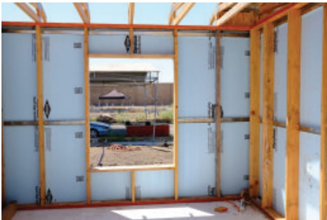
Fig. 5.4 Exterior wall studs set 24" on center
