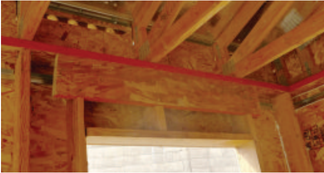
Fig. 5.7 Removable headers reduce insulation gaps The header is installed with screws. Then it is removed temporarily by insulators, so they can insulate the cavity behind.
