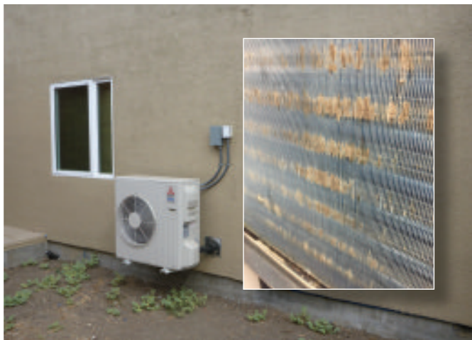
Fig. 10.6 Outdoor HVAC unit and sawdust-clogged fins
