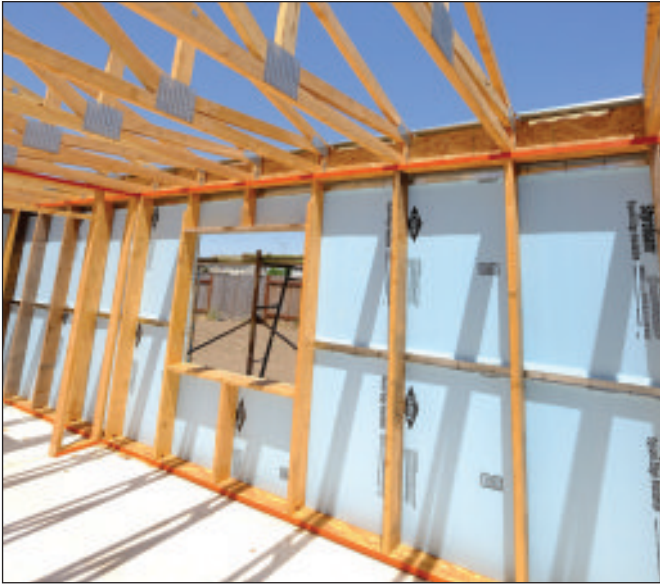
Fig. 6.2 Exterior wall studs 24 in. on center, aligned under framing above
