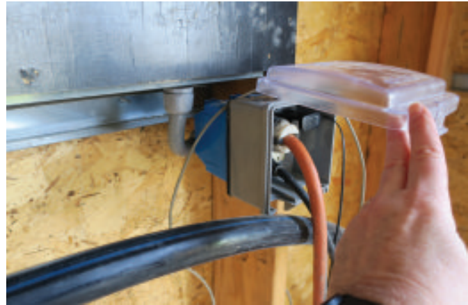
Fig. 9.2 Construction power from a splitter panel
