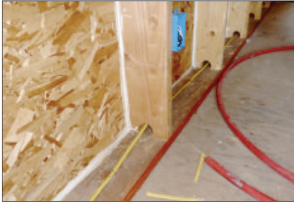
Fig 6.17 Stud bases pre-drilled or notched for wiring
