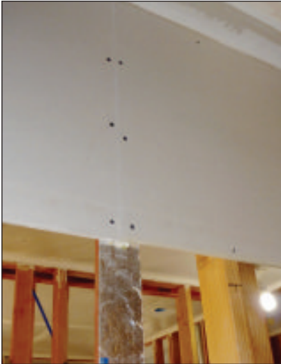
Fig. 5.20 Horizontal drywall with OSB-backed splice Rather than landing on a stud, the sheets are spliced and backed securely using OSB off-cuts, saving a surprising amount of wall board.
