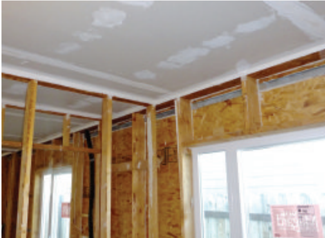
Fig. 5.12 The right time to find and fix air leaks
