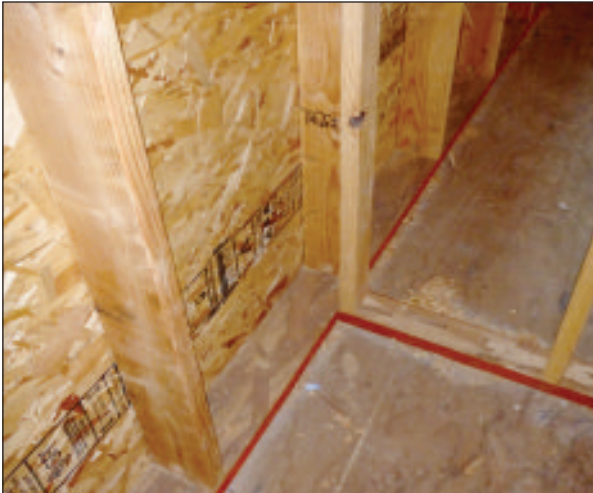
Fig. 6.5 Frame to minimize interference with batt insulation
