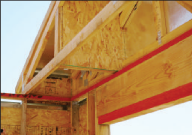
Fig 6.15 Ground-assembled gable end trusses
