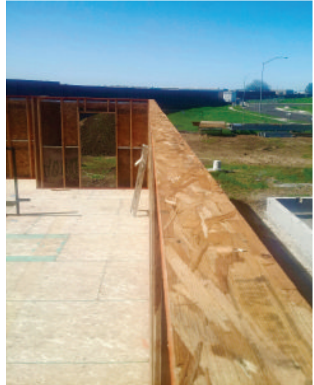
Fig. 5.4 Single LSL top plate: 36 ft. long
