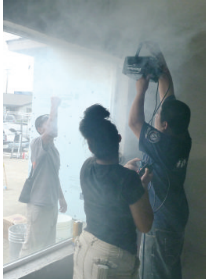
Fig. 5.13 Use a theatrical fog generator to find leaks
