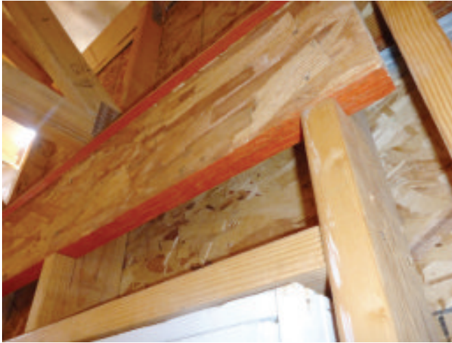
Fig 6.12 Removable header
