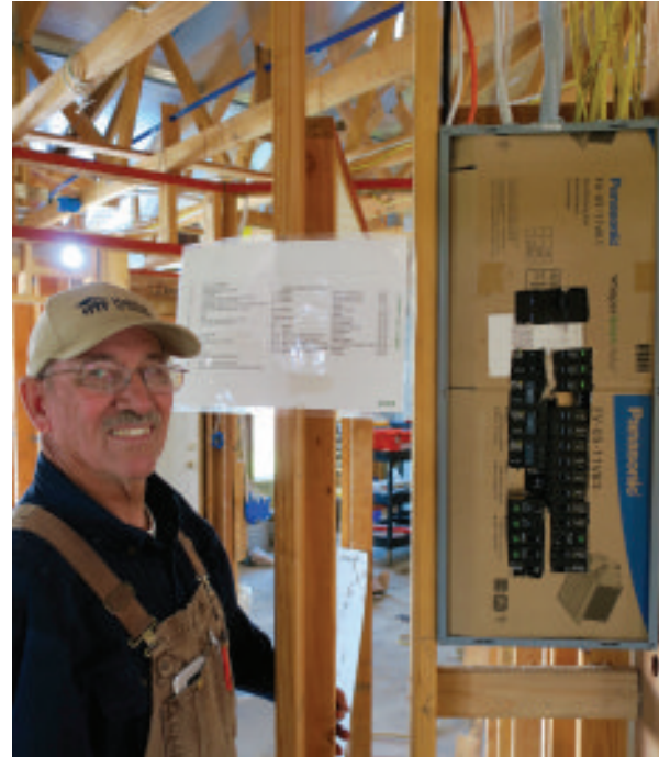
Fig. 9.3 Wire jacket color indicates the circuit's amp rating
