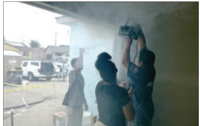
Figure 1.3 - In-process verification. For example, the fog machine Achieving profitable market-rate ZNE homes demands new patterns of workflow, supported by new tools. Some of these tools are expensive and unfamiliar. But big improvements come trusting workers (and requiring them) to test and measure the results of their work, as they work. In this photo, a blower door is used to positively-pressurize the building. Then a fog machine generates fog inside, and is held near suspect joints. From outside, the worker can locate air leakage points by the escaping fog. Then those can be sealed up, immediately. From the immediate reduction in air flow through the blower door, air tightness is measured in real time—instead of long after the crew has left the job and it’s too late to seal the leaks.
