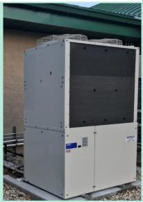
For heating-dominated climates, the GHP's high heating efficiency has the potential to reduce energy costs, offsetting the cost premium of the equipment. Heat recovered from the engine is used to supplement heat output and maintain supply temperatures without any backup heating.
