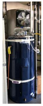
tank. Combined with internal heat recovery, this maintains hot water capacity and temperatures while using significantly less natural gas. Vapor absorption heat pump cycles like this have been used for decades, but only recently have been applied to residential water heating.
