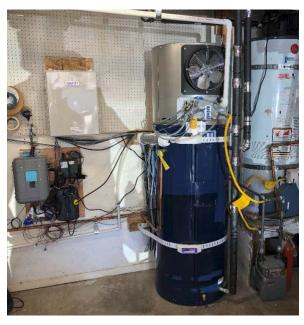
The GHPWHs were monitored over a period of approximately 12 months, with some downtime to allow for adjustments and repairs. The estimated annual energy savings of gas totaled 36%. This modest savings mirrors the relatively modest hot water usage at the home, well under the average seen across the other homes in this study. The homeowner indicated that the hot water supply was better with the GHPWH than their previous water heater and their overall experience with the GHPWH as excellent.
