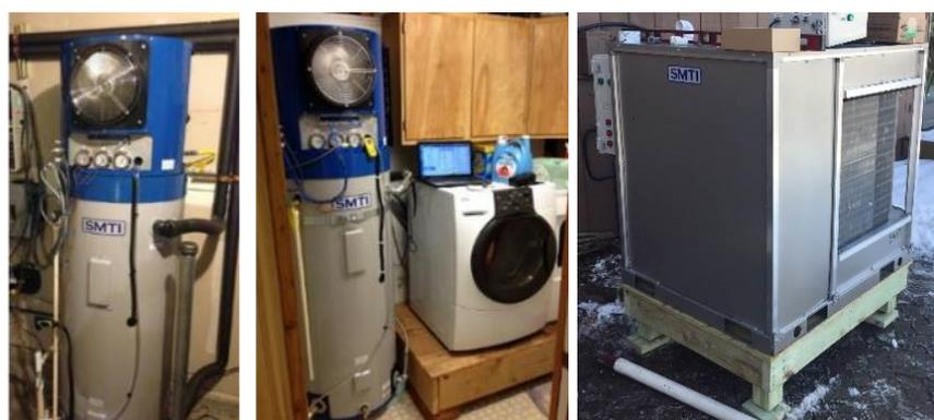
**Figure 5 Photos of DHW-Only GAbHP and GAbHP Combi Systems in Field Trials**
