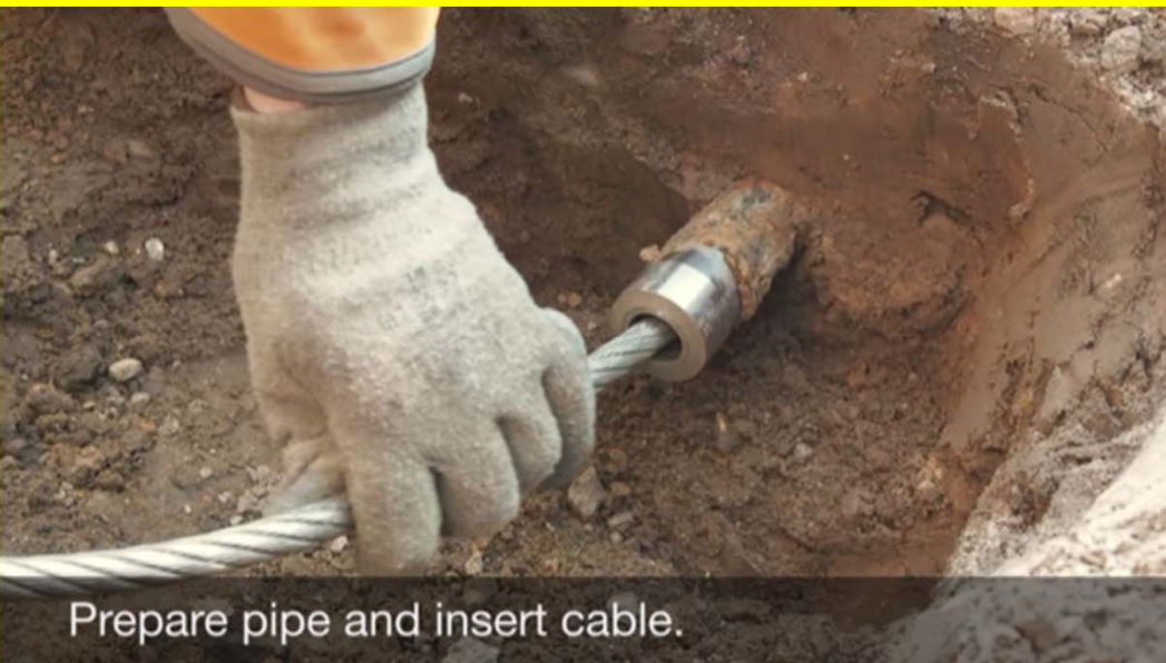
Prepare pipe and insert cable.
