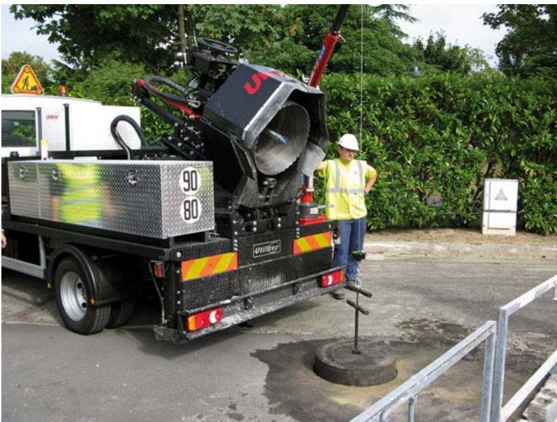
Fig. 2: Corina and reinstatement process – establishing the core bore.
