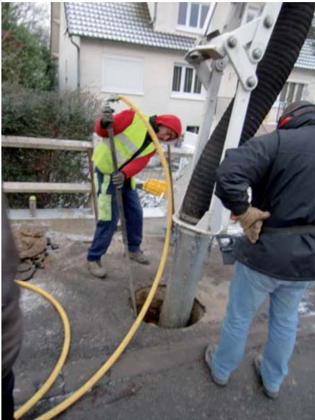
Fig. 3: Application of a suction excavator.
