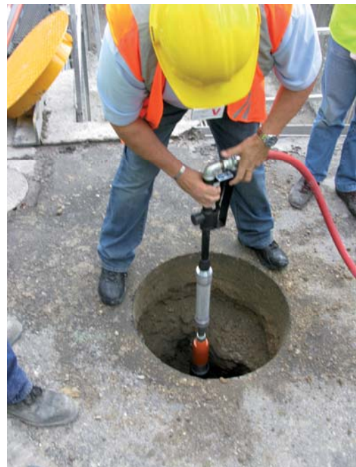
Fig. 5.1: The bore core is re-instated.
