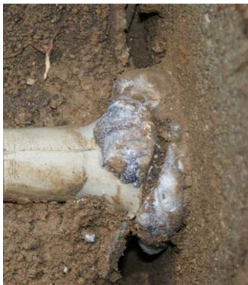
Fig. 7.1: Exposed wall duct
