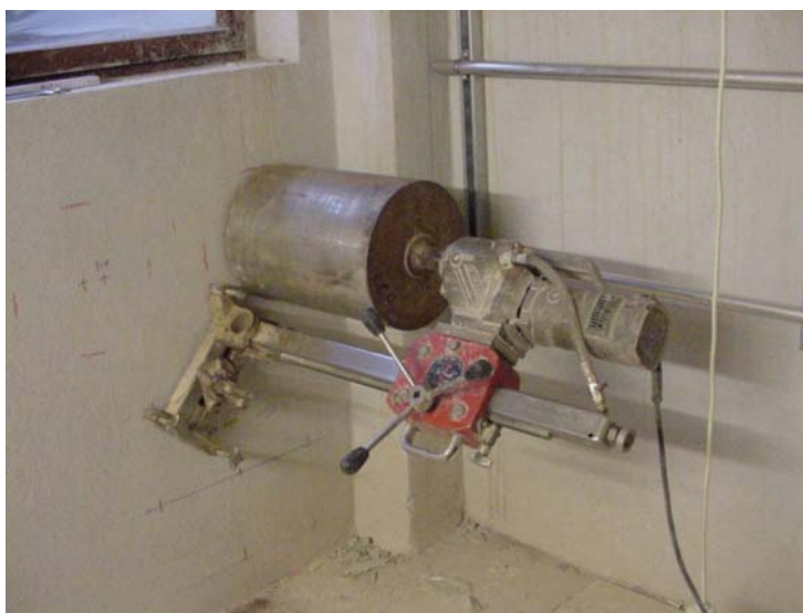
Fig. 7.2: Core bore in the building's basement.
