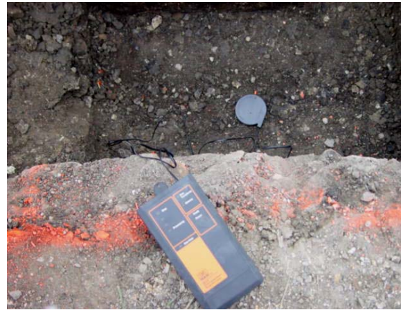
Figure 3 - Soil Compaction Supervisor
