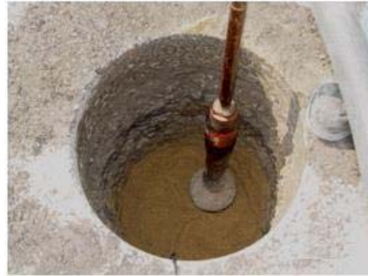
Figure 1- Use of "jumping jack" to compact backfill in keyhole
