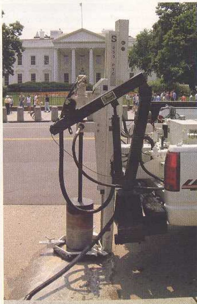
A core-hole cutter makes small street cuts efficiently.
