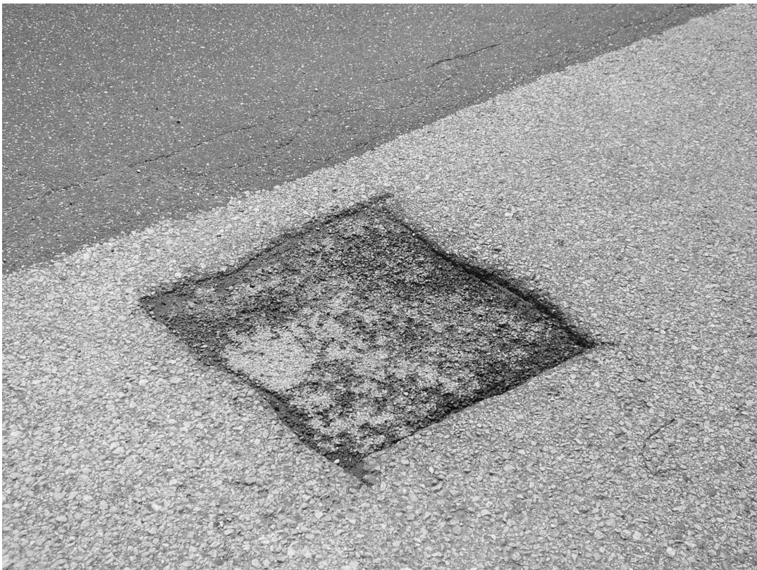
Figure 4: Traditional street cut after four years
