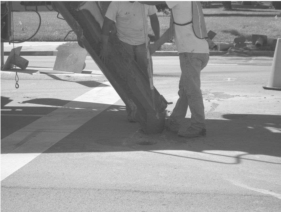
Figure 3: Flowable fill backfill being placed in core hole
