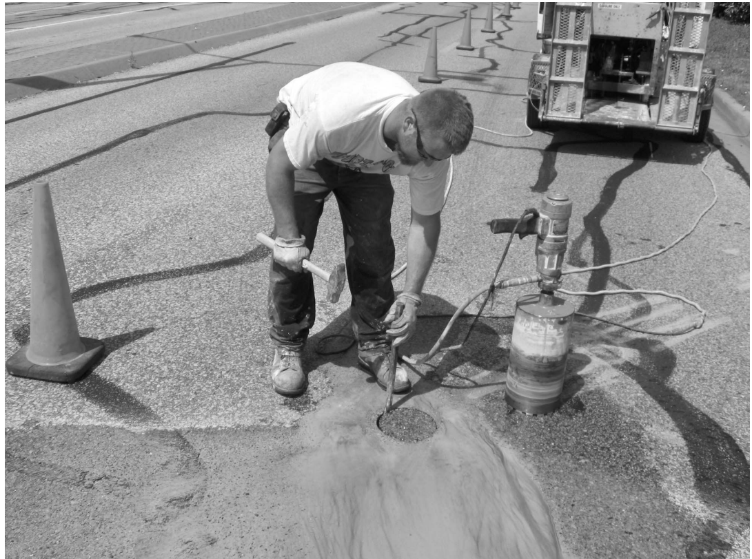
Figure 2: Core being manually extracted
