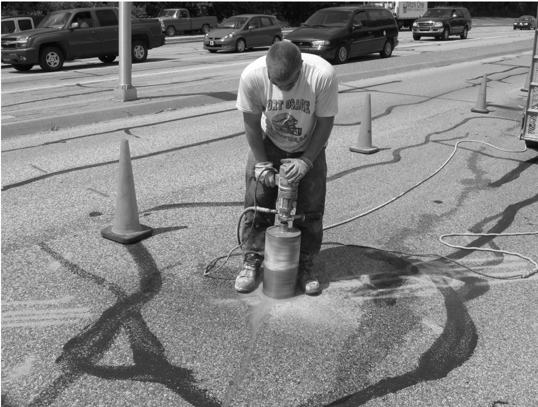
Figure 1: Core being cut with manually operated drill
