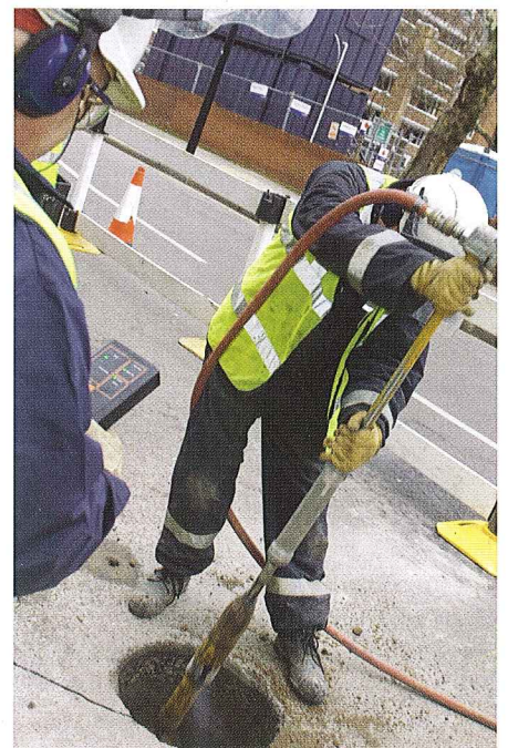
An engineer fixing a gas main using long-handled tools.
