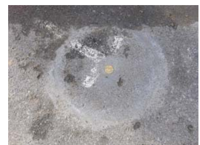
10. Reinstated core – almost invisible
