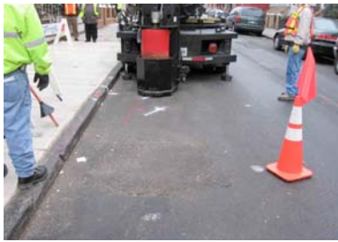
1. Coring unit with conventional repair in foreground
