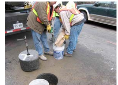
8. Mixing the Utilibond
