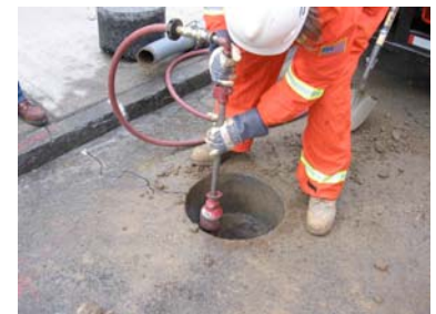
7. Compaction (note wire from soil compaction supervisor)
