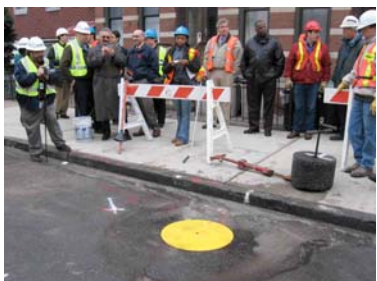
4. Temporary road plate
