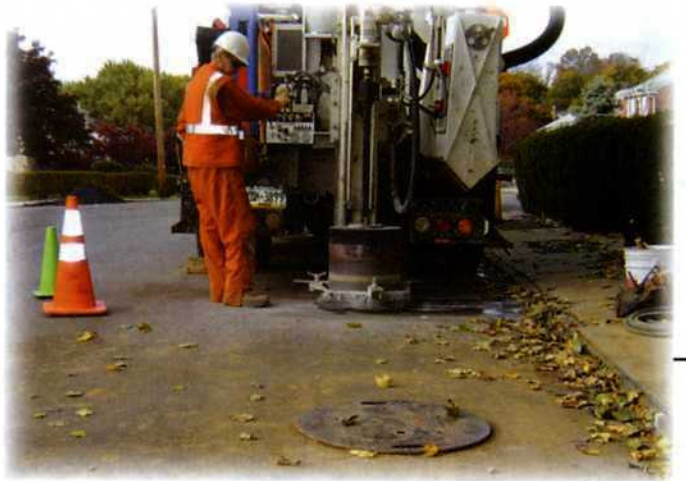
Coring the street
