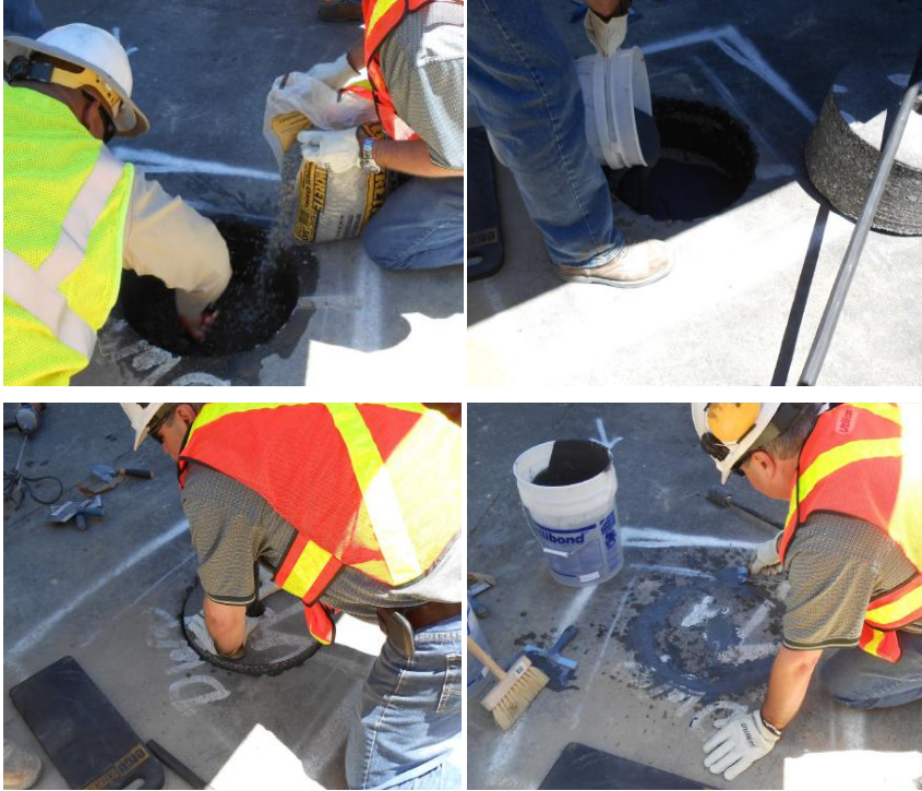
Replacing the pavement core for a permanent roadway restoration
