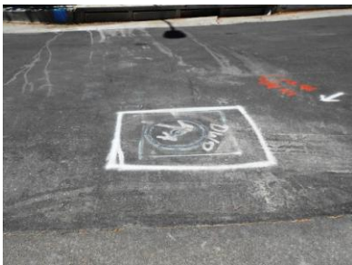
Restored pavement core open to traffic after 30 minutes
