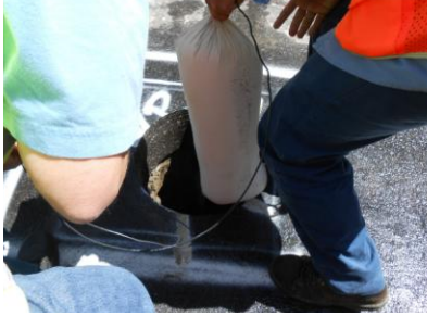
Anode being installed in the excavation below the steel water main
