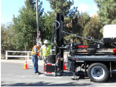
Coring the pavement to expose the steel water main
