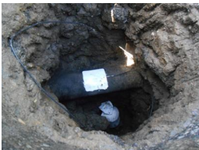
Anode installed in keyhole and coating replaced on pipe
