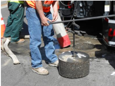
Extracting the 18" diameter core from the pavement
