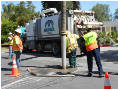
Vacuum excavating to expose the steel water pipe
