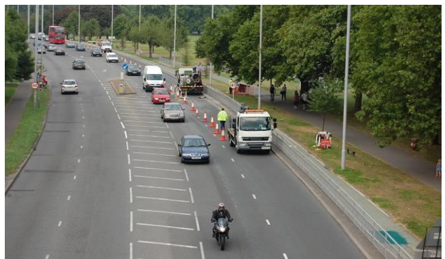
'Core & Vac' operation
