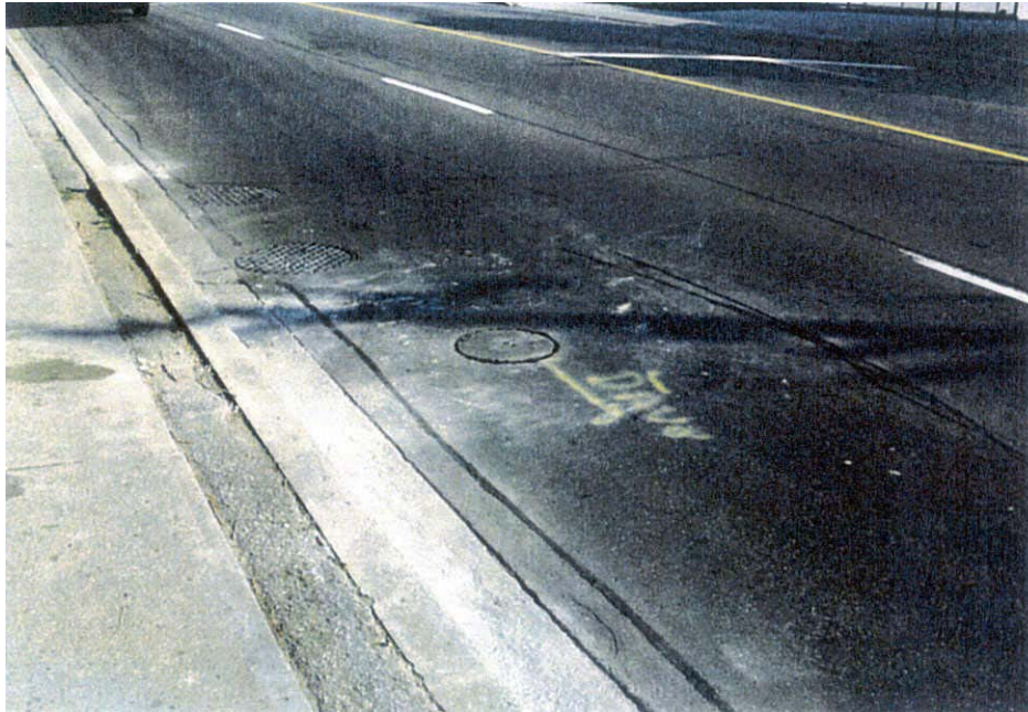
Photo 3 – View of reinstatement in two weeks after installation in 1995.
