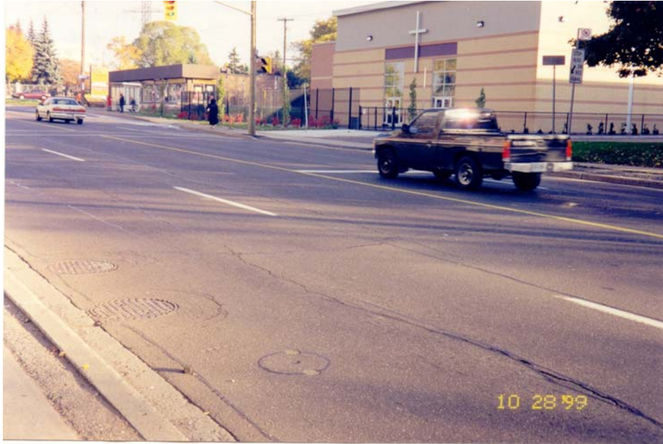
Photo 6 – Kennedy Road reinstatement in October 1999.
