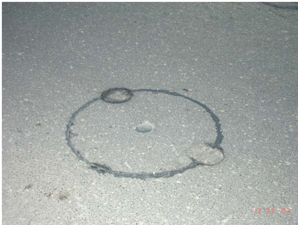
Photo 9 – Close view of Kennedy Rd. reinstatement in December 2002.
