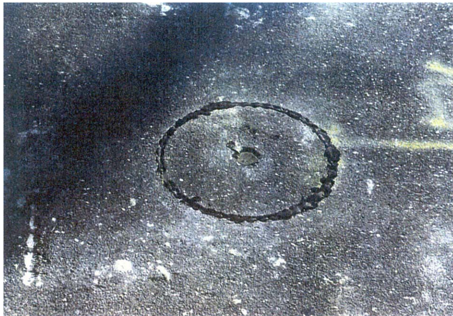
Photo 4 – Close view of reinstatement two weeks after installation in 1995.
