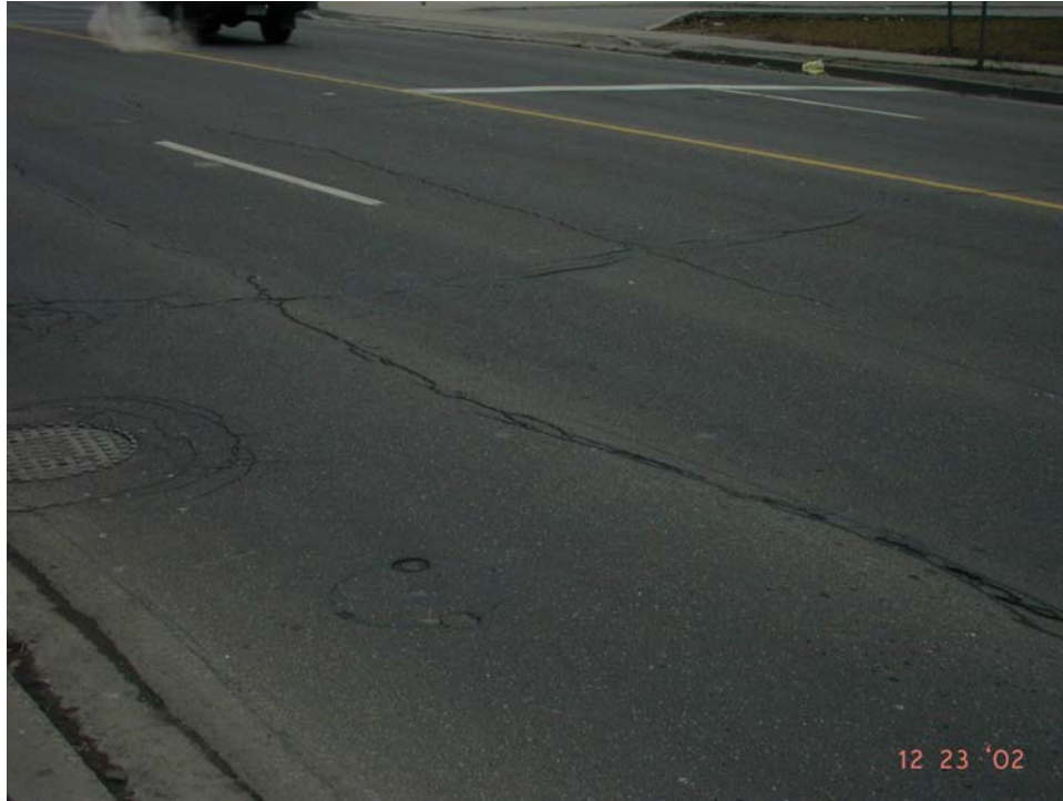
Photo 8 – Kennedy Rd. reinstatement in December 2002.
