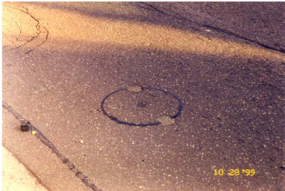
Photo 7 – Kennedy Road reinstatement in October 1999.
