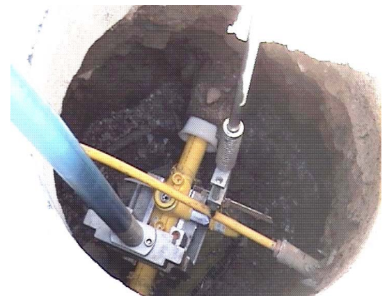
Electrofusion of service tee onto main.
