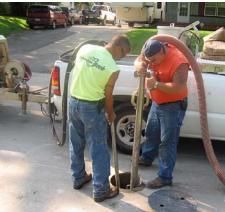
Vacuum excavating and sandblasting.
