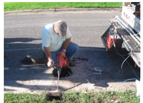
Wires run to a test station via a groove sawed in the concrete and a hole drilled through the curb.
