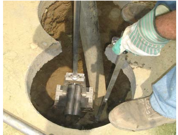
Above: Keyhole Installation of Mueller 2" Full Seal Repair Clamp
