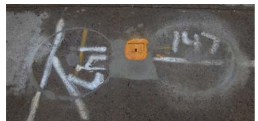
Two 18-inch-diameter holes were cored to allow to access the steel gas main and service.
