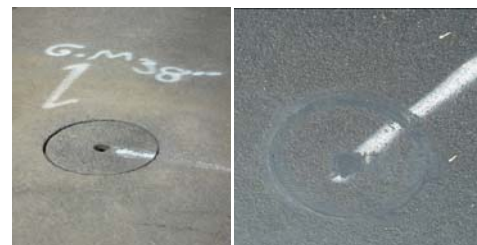
Completed STM/Keyhole location.
