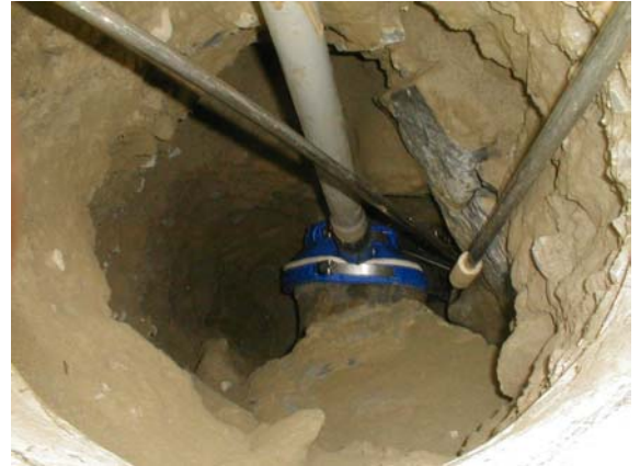
Keyhole installation of Permabond repair system
