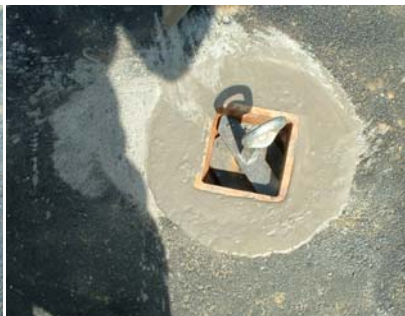
Grout is poured up to surface of existing pavement.
