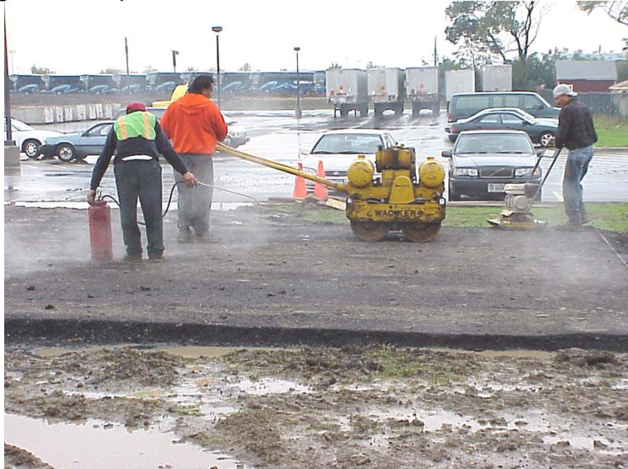
Figure 36. Construction of the asphalt layer in the outdoor test section
