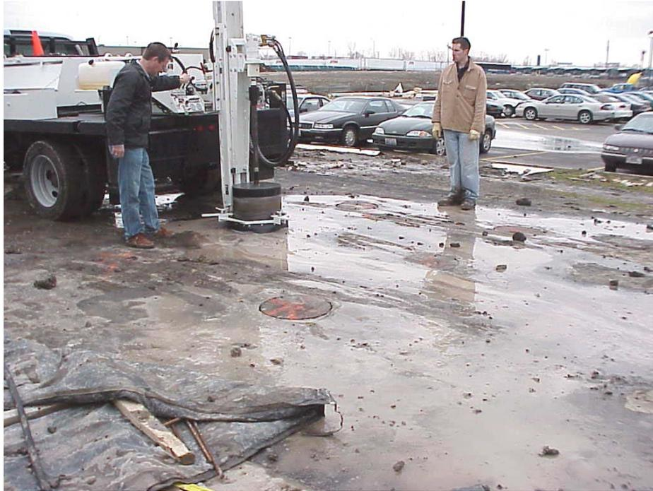
Figure 37. Drilling the 18-inch cores using the “SIMCO” Drilling machine
