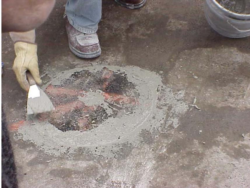
Figure 41. Scooping out the excess grout after core placement.
