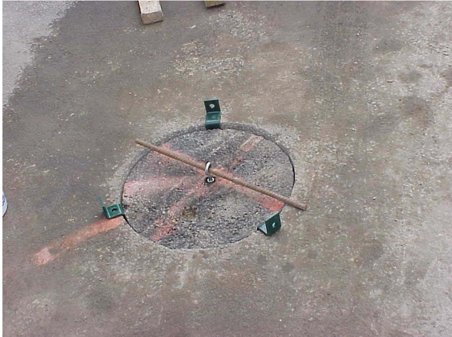
Figure 38. Pre-marking and anchoring the core
