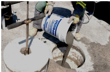
Figure 4. Utilibond is safe and easy to use – just add water, mix and pour into hole.
