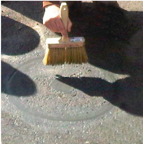
Keep surface wet to prevent premature hydration.
