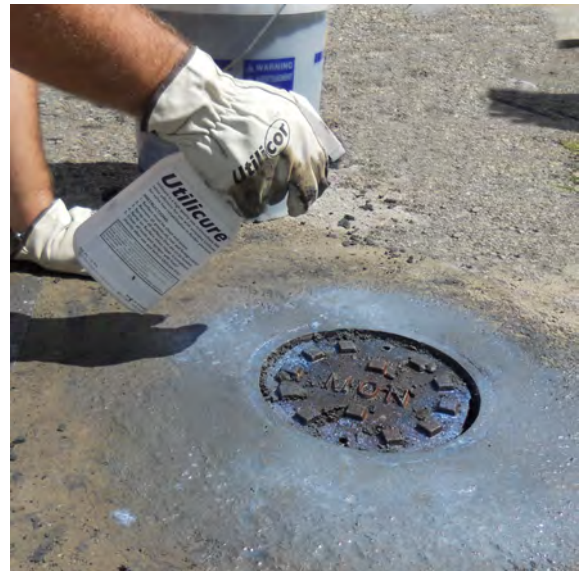
Utilicure being applied to reinstated valve box.
