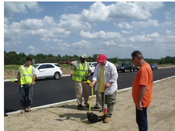
gas water and sewer located
