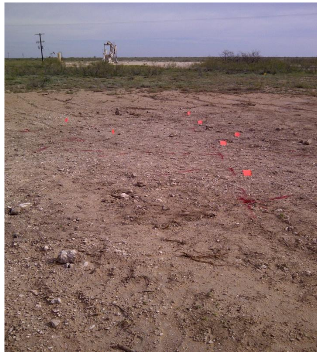
crossing pipes in test field
