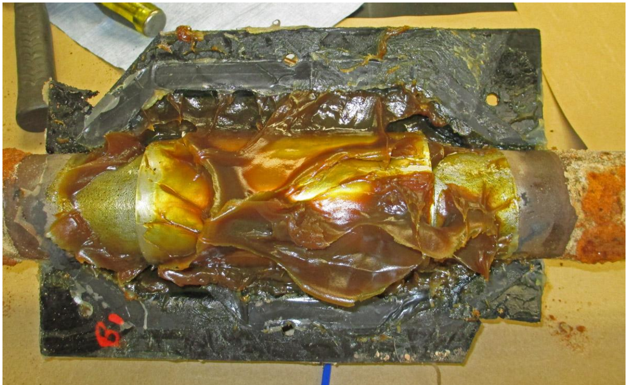
Figure 7 After partial removal of enclosure and wax
