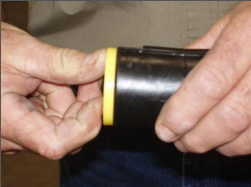
INSTALL THE ELECTROFUSION COUPLING OVER THE STACK OF THE ALDYL-A TEE UNTIL IT BOTTOMS ON TEE OUTLET.
