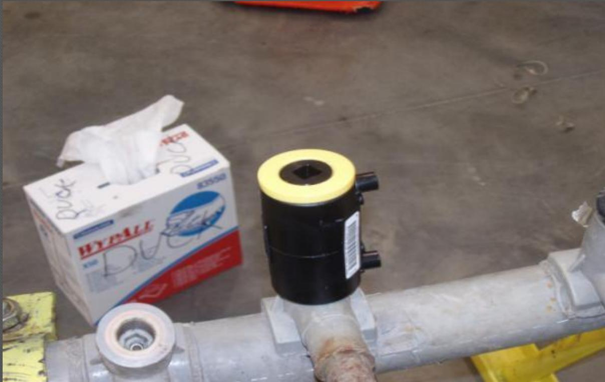
This completes the Aldyl-A Repair Kit assembly process. Test the finished assembly per company procedures. (i.e. soap test entire fitting)
