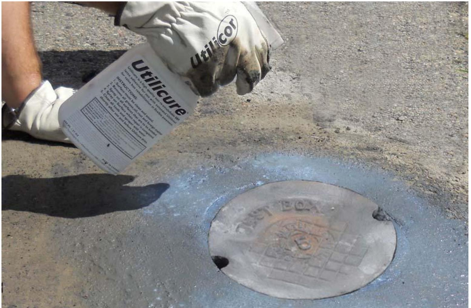
Spray surface with Utilicure to ensure proper hydration and Prevent surface cracks.
