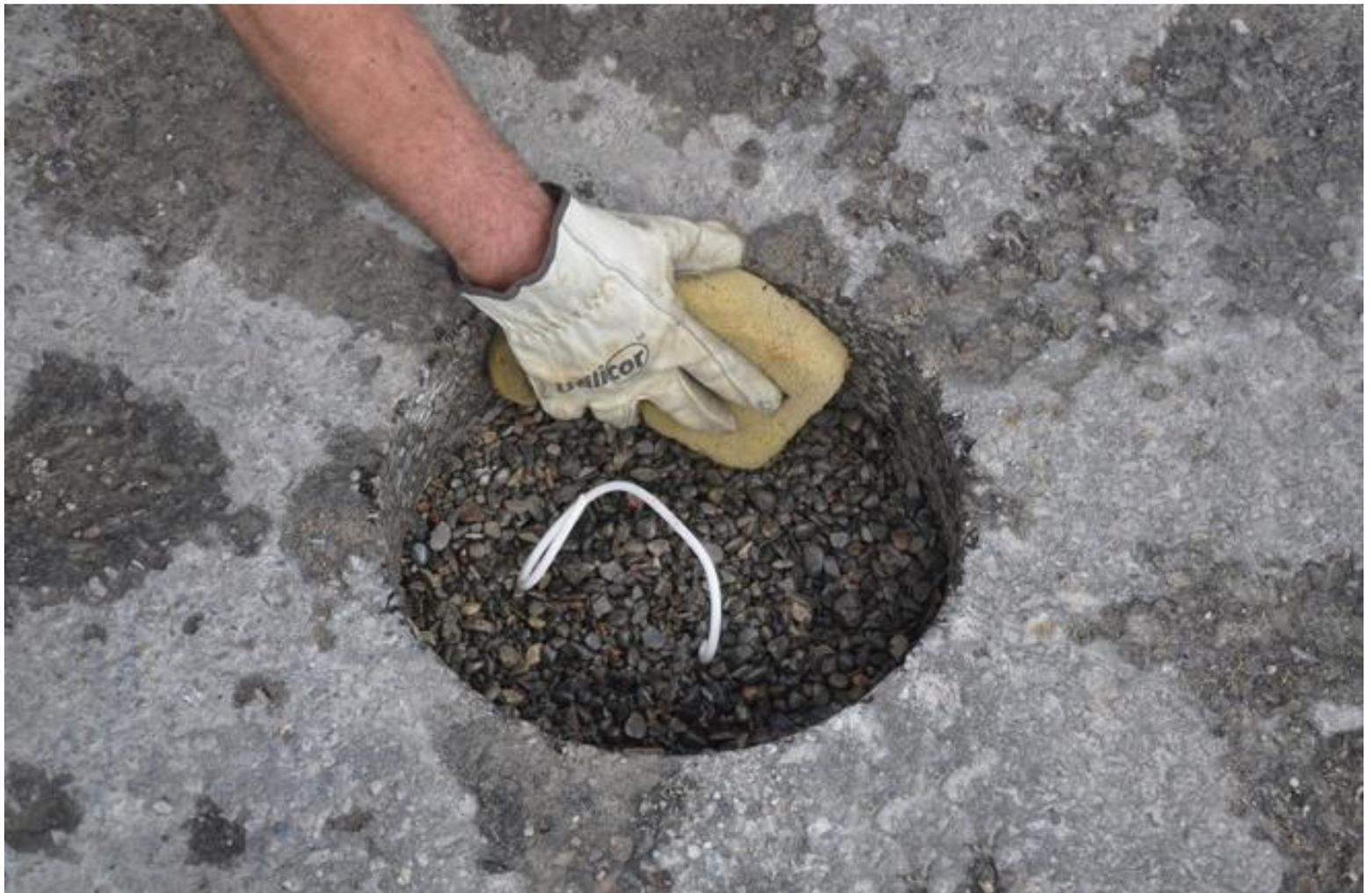
After test wire is installed and hole is back filled and compacted to about 2 inches below base of pavement or 6 to 8 inches below the surface clean the sides of the pavement.
