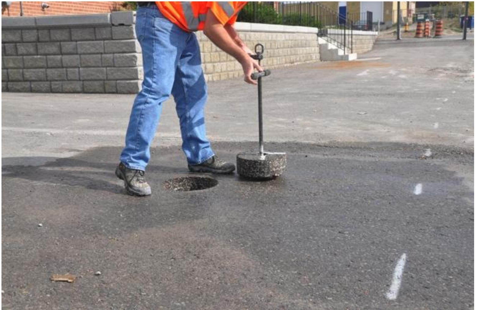
Remove core with core puller and or sunken valve box by hand. Clean up area.
