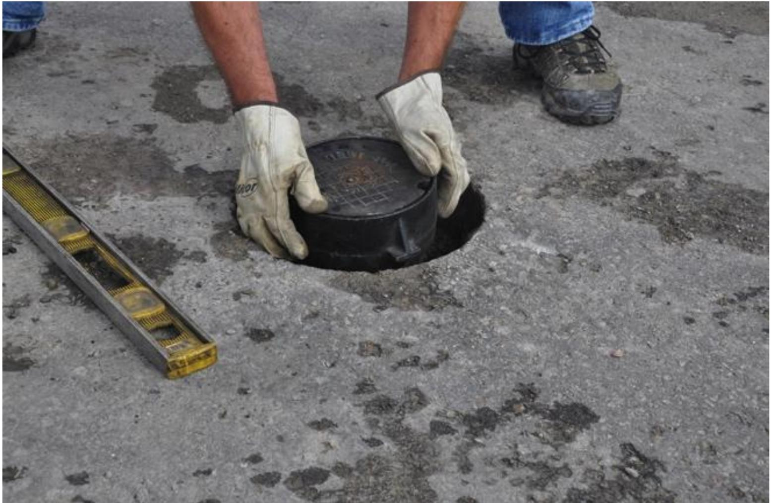
Add 1-2 inches of pea stone and install test box or new valve box.
