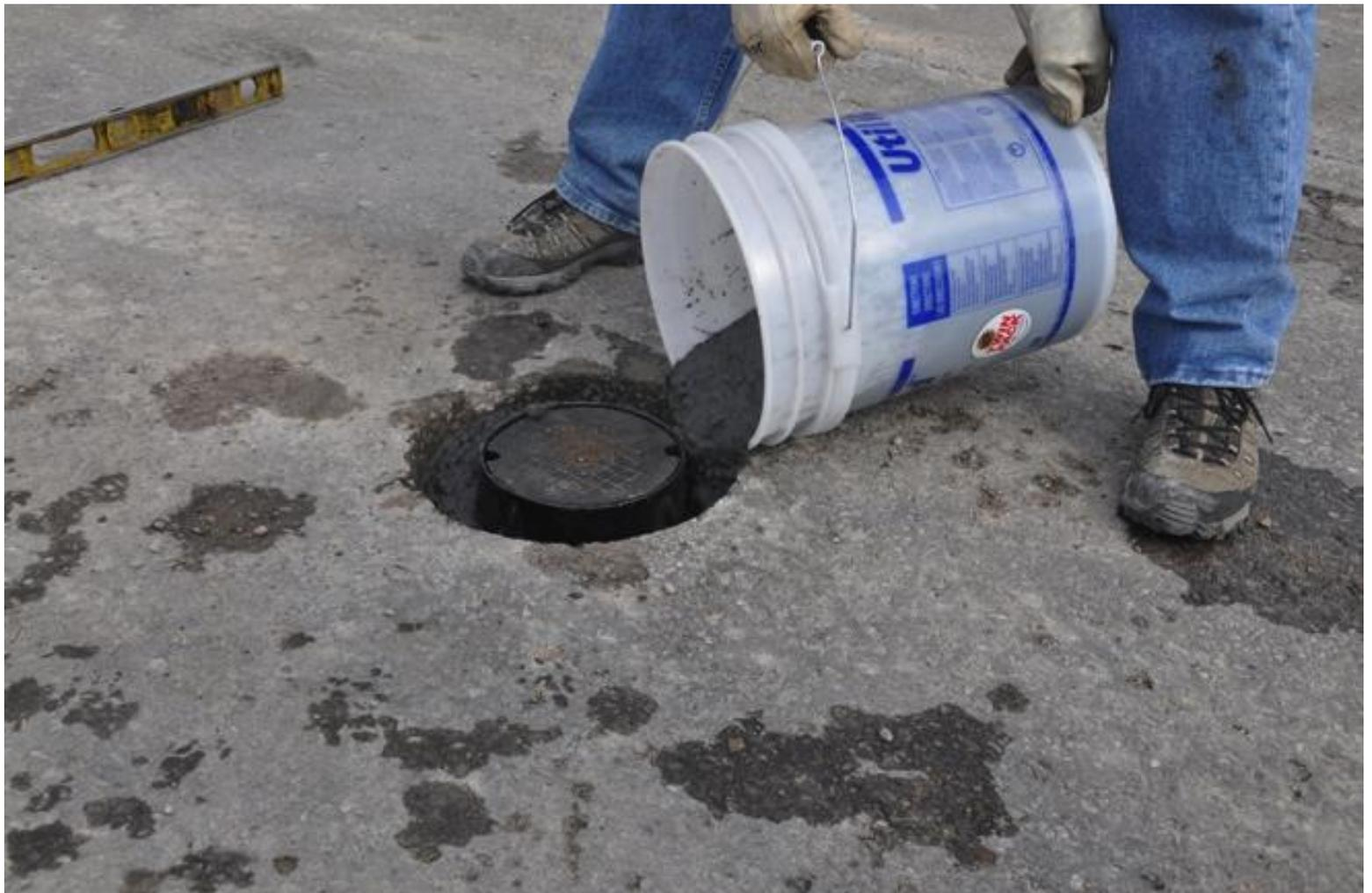
Carefully pour mixture into the hole around the valve box.
