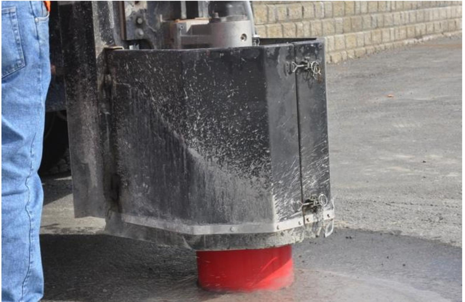
Core 12" hole through pavement around existing valve box (remove pilot pit) or location of test station.
