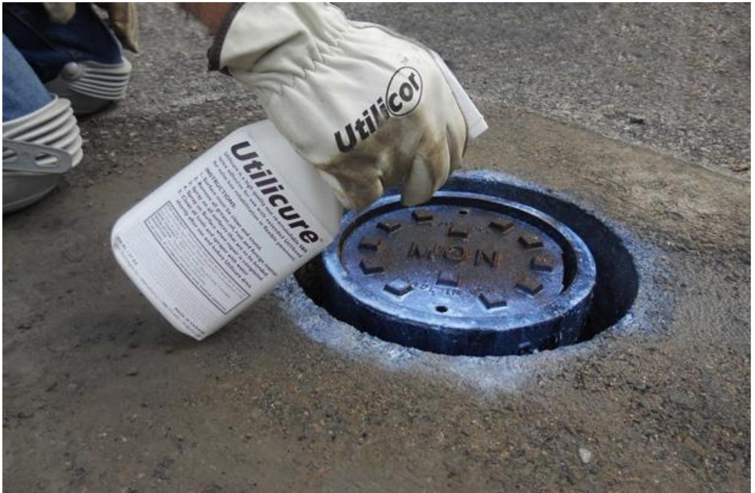
Generously spray all areas to be bonded, on valve box and pavement with Utilicure. Do not allow Utilicure to dry, if it does reapply.
