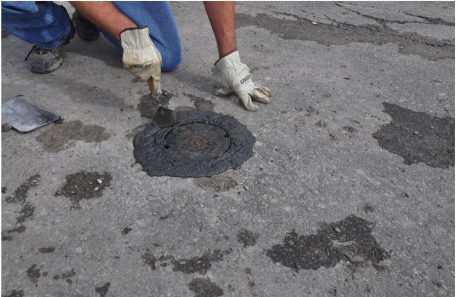
Consolidate the mixture into the hole to make sure there are no voids. If the Utilibond mixture is slightly below the surface add pea stone to mix and consolidate again.
