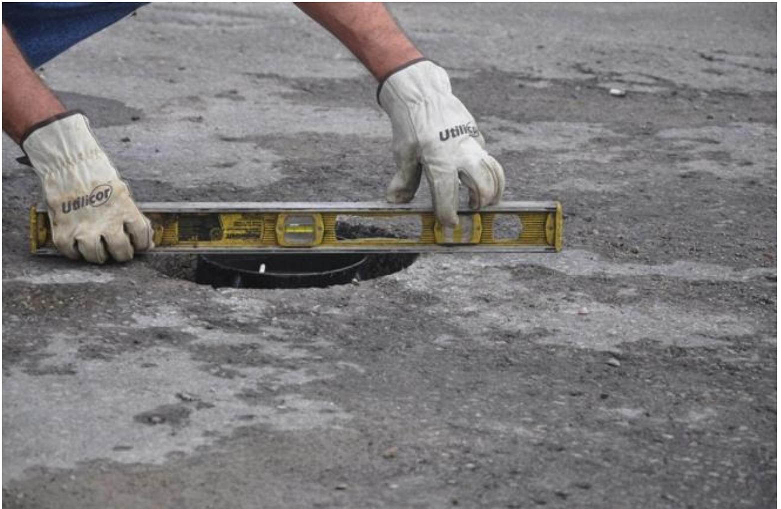
Using a straight edge make sure the top of the box is flush with the surrounding pavement.
