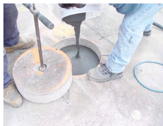
Utilibond poured into hole
