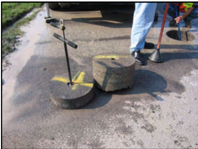
Above: The core has been extracted from the roadway, but in two pieces. This core has delaminated.
