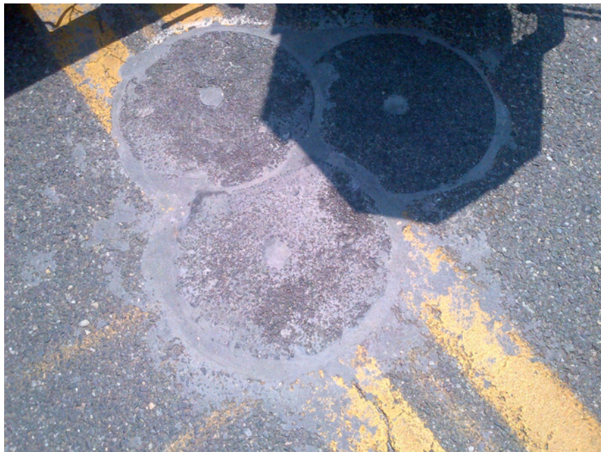
As seen above, a triple core cut, extracted, and reinstated as one repair
