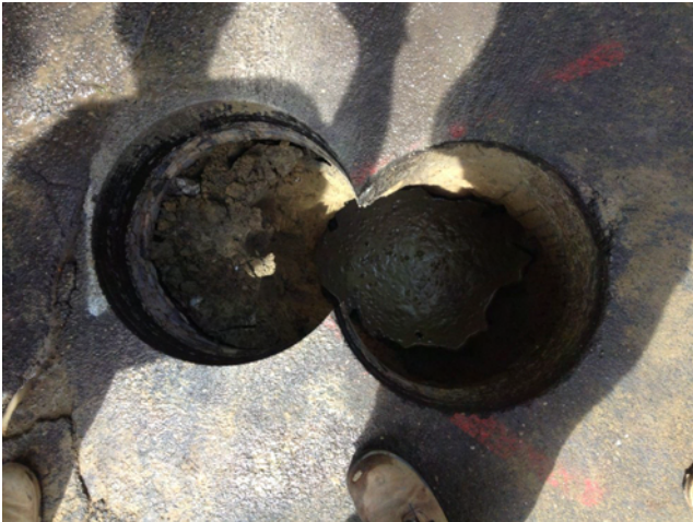
Two 18" diameter cores are cut to allow for greater access to buried facility
