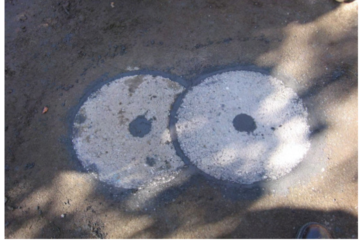
Two cores that have been simultaneously reinstated
