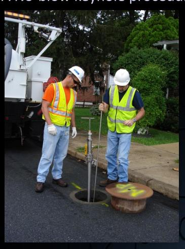
A special threaded plug is installed into the steel main.
