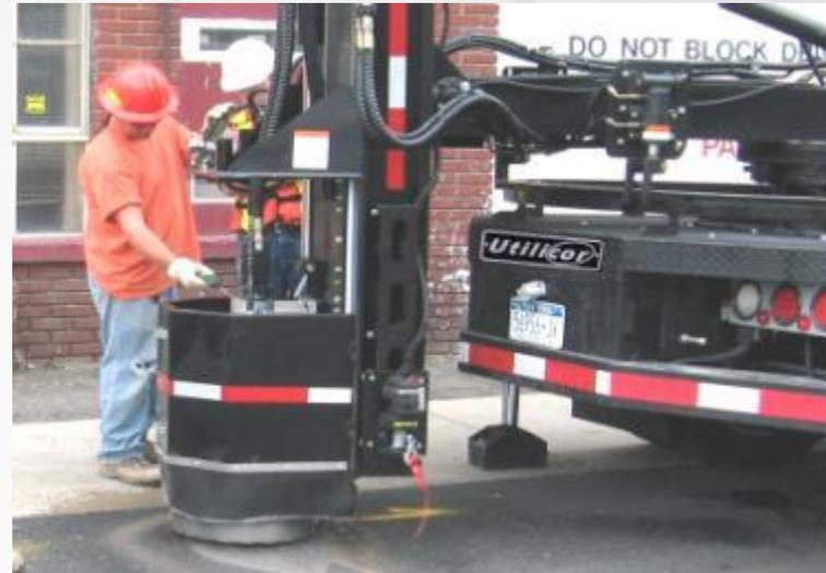
The precise coring process when combined with vacuum excavation reduces loading adjacent to the excavation and **minimizes or eliminates any zone of influence.**
