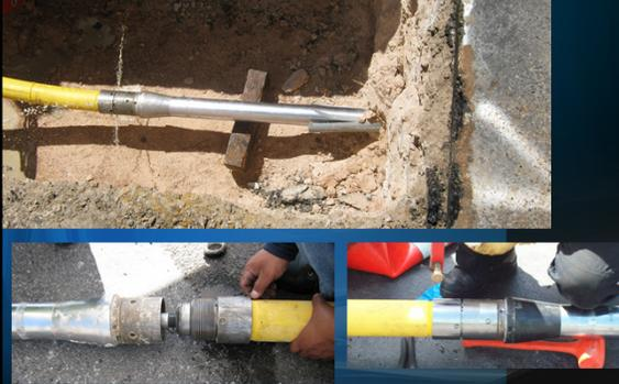
Two photographs showing the pipe installation. The top photo shows a yellow and silver pipe being pulled through a trench. The bottom photo shows workers at the surface connecting sections of the pipe.
