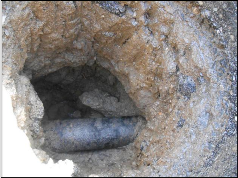
Exposed 6" steel water pipe
