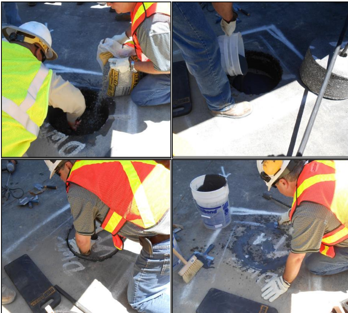
Replacing the pavement core for a permanent roadway restoration
