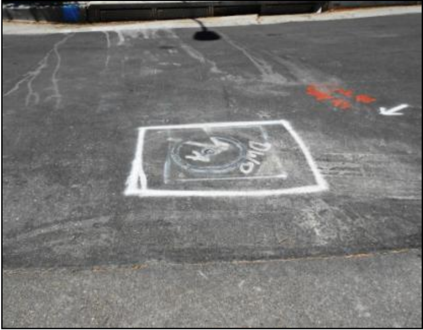
Restored pavement core open to traffic after 30 minutes
