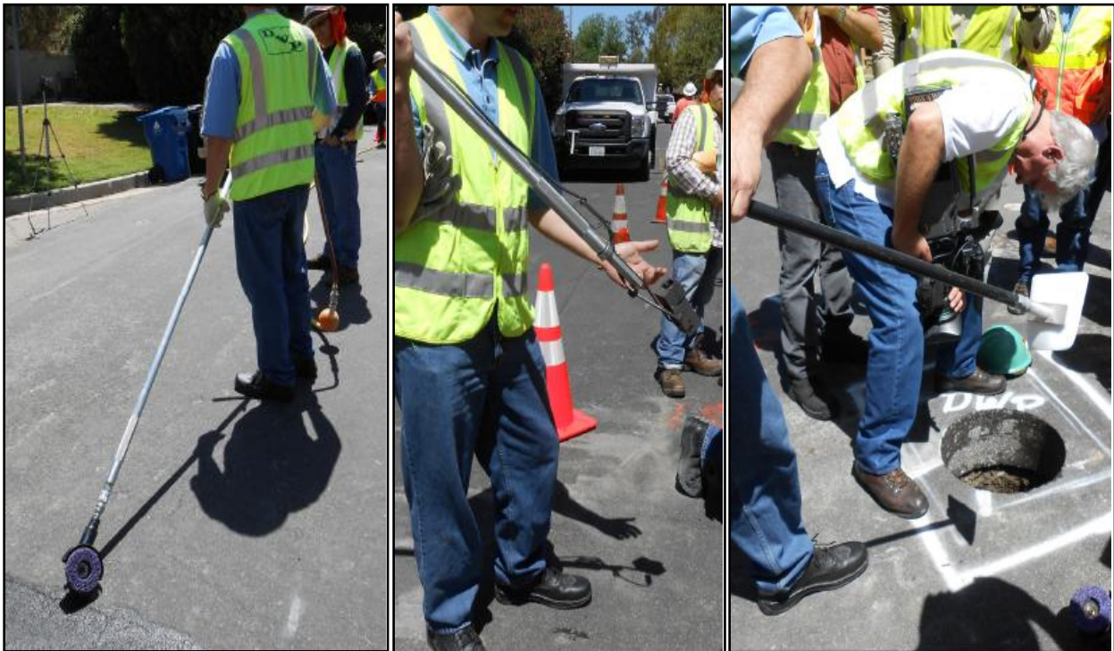
Long-handled tools used to grind away the pipe coating, cadweld the wire to the pipe, and re-coat the pipe and exposed wire
