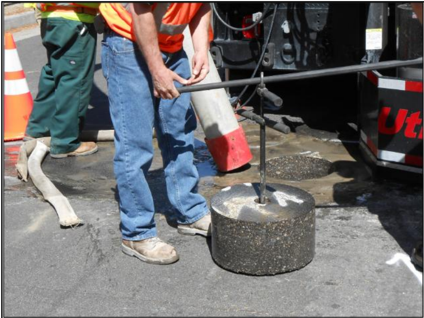
Extracting the 18" diameter core from the pavement
