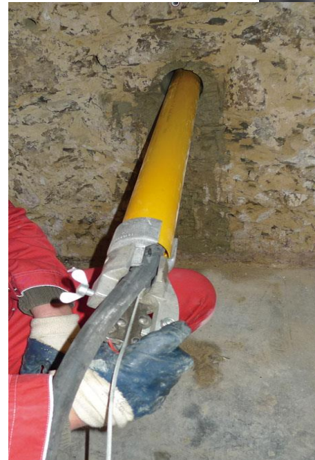
Removing of the host pipe
