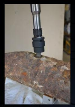
After the pipe plug has been successfully started into the main the plug is tightened using the pipe plug socket on the <sup>3</sup>/<sub>4</sub>" drive extension.
