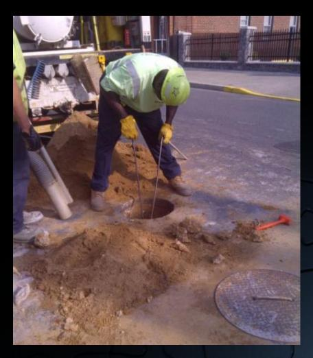
Core cut 18 inch diameter openings demand that all operating procedures are thoughtfully designed and performed using professional tooling
