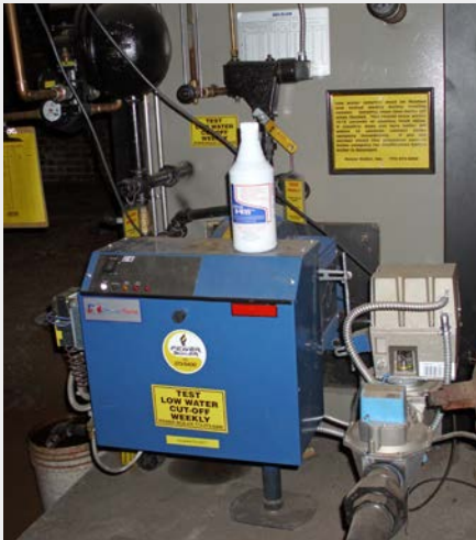
Retrofit measures included a new boiler.
