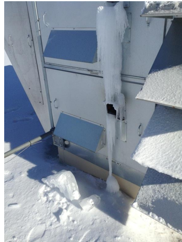
Big Box Retail Store Condensing DOAS Flues in MN
