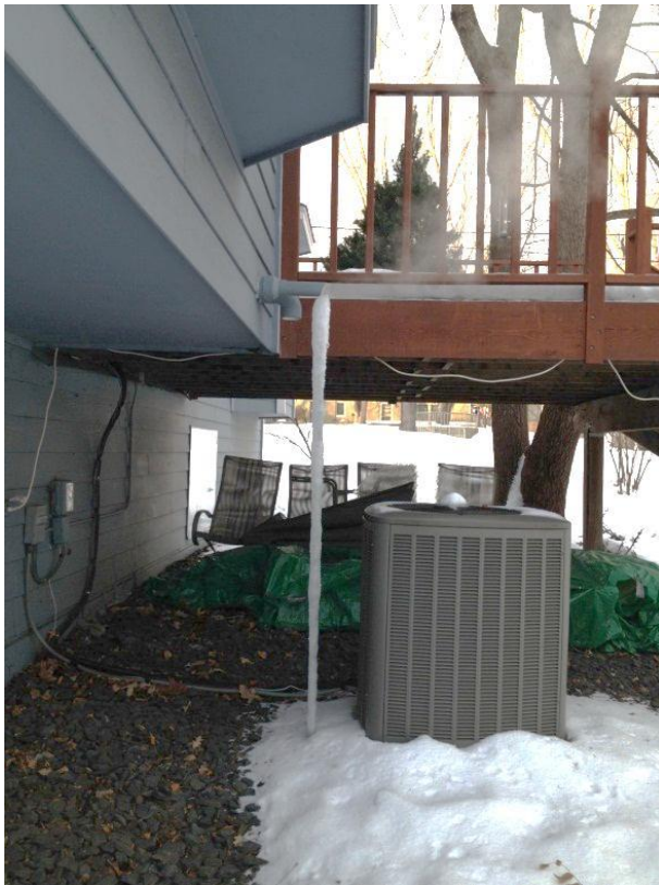
Residential Condensing Furnace Flue in MN
