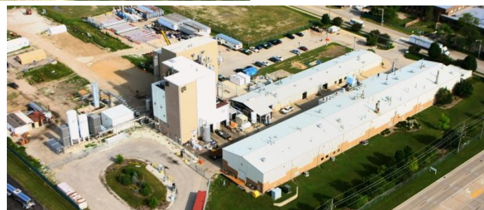
Energy & Environmental Technology Center
