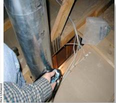
Without effective insulation, these ducts waste the HVAC equipment's capacity by heating and cooling the crawl space. Imagine the savings potential.
