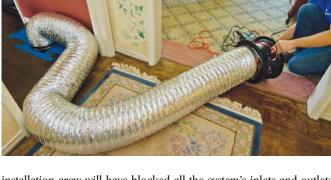
installation crew will have blocked all the system's inlets and outlets and connected the system to a calibrated fan. That fan pressurizes the system and measures any outward air flow. While the fan keeps the system under positive pressure, the crew keeps finding and sealing cracks, drill holes and seams until the calibrated fan shows that the system's air leakage is nearly zero.
