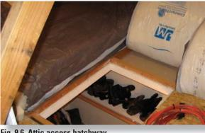
Fig. 9.6 Attic access hatchway
