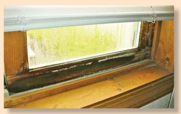
**Fig. 10.2 Extensive frame damage - Consider replacement** Single-pane glass stays cold during winter weather, which can lead to condensation and damage, in addition to high heating bills.
