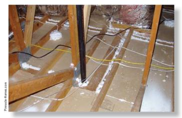
Fig. 9.13 Sealing the top plates of interior walls and the seams of ceiling gypsum board panels with spray foam Also note the foam-covered, air-sealed electrical box
