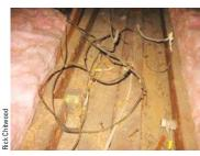
Fig. 3.9 Wiring deficiencies like this one are a fire hazard, and *must* be corrected before filling the attic with insulation
