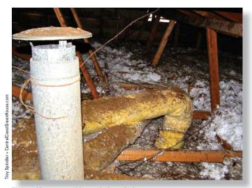
**Fig. 2.7 Unexpected hazards in existing systems** *This furnace vent stack terminates in the attic, just above the children's room. Products of combustion, among them deadly carbon monoxide gas, can drift down into the home.*
