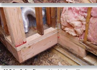
**Fig. 9.2 Before & after - Fix any moisture intrusion problems** *Fix any moisture problems before air sealing begins. If you don't... you'll increase moisture problems by air sealing the building.*
