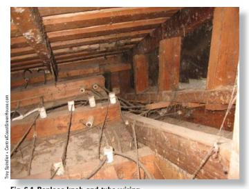
**Fig. 6.4 Replace knob-and-tube wiring** With knob-and-tube wiring it's not safe to properly insulate the attic. Old wiring connections heat up under insulation, creating a fire hazard. Replace such wiring with modern, code-compliant electrical work before covering it with insulation.
