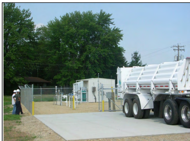
Figure 33: Agri-Waste RNG Transfer Station with Tube Trailer in Emerald, WI.
