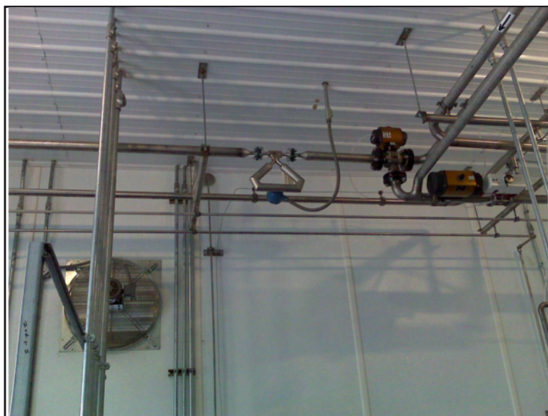
Figure 41: Mass Flow Meters at Emerald Dairy in Emerald, WI. From left to right: Coriolis mass flow meter, thermal mass flow meter.
