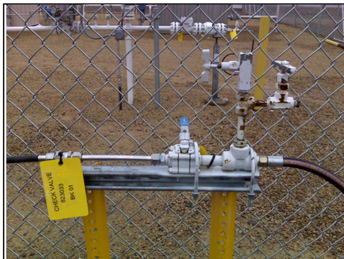
Figure 34: Biogas injection port into the transmission line at Northern Natural Gas facility in Baldwin, WI.
