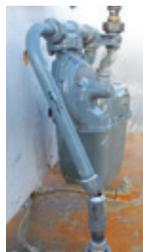
A breakaway fitting to enhance gas system safety is a low-cost option to reduce risk to aboveground Meter Set Assemblies (MSAs) when impacted by outside forces, such as vehicular impact. The breakaway fitting being commercialized by OPW can be installed directly to new and existing meter sets to stop the flow of gas when impacted and reduce the risk of a leak, fire, explosion, and/or property damage. Field testing at several U.S. utilities received very positive feedback.
