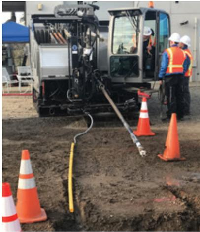
GTI partnered with PG&E to bring pre-commercial Optimized Radar to Find Every Utility in the Street (ORFEUS) technology to the U.S. for live field evaluations. The real-time radar obstacle detection system for horizontal directional drilling (HDD) was developed in Europe with funding support from the European Union.
